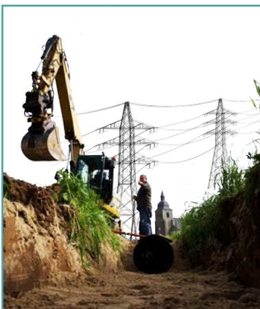
We also need to move some of the underground gas pipes and overhead electricity cables.
