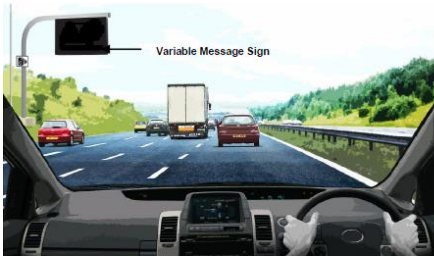
Figure 4b: Illustrative smart motorway scheme section operating in normal motorway conditions with a blank cantilever mounted variable message sign
