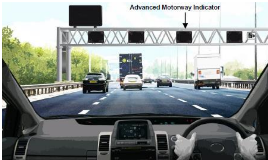
Figure 4a: Illustrative smart motorway all-lane running scheme section operating in normal motorway conditions with blank advanced motorway indicators and blank gantry mounted variable message sign
